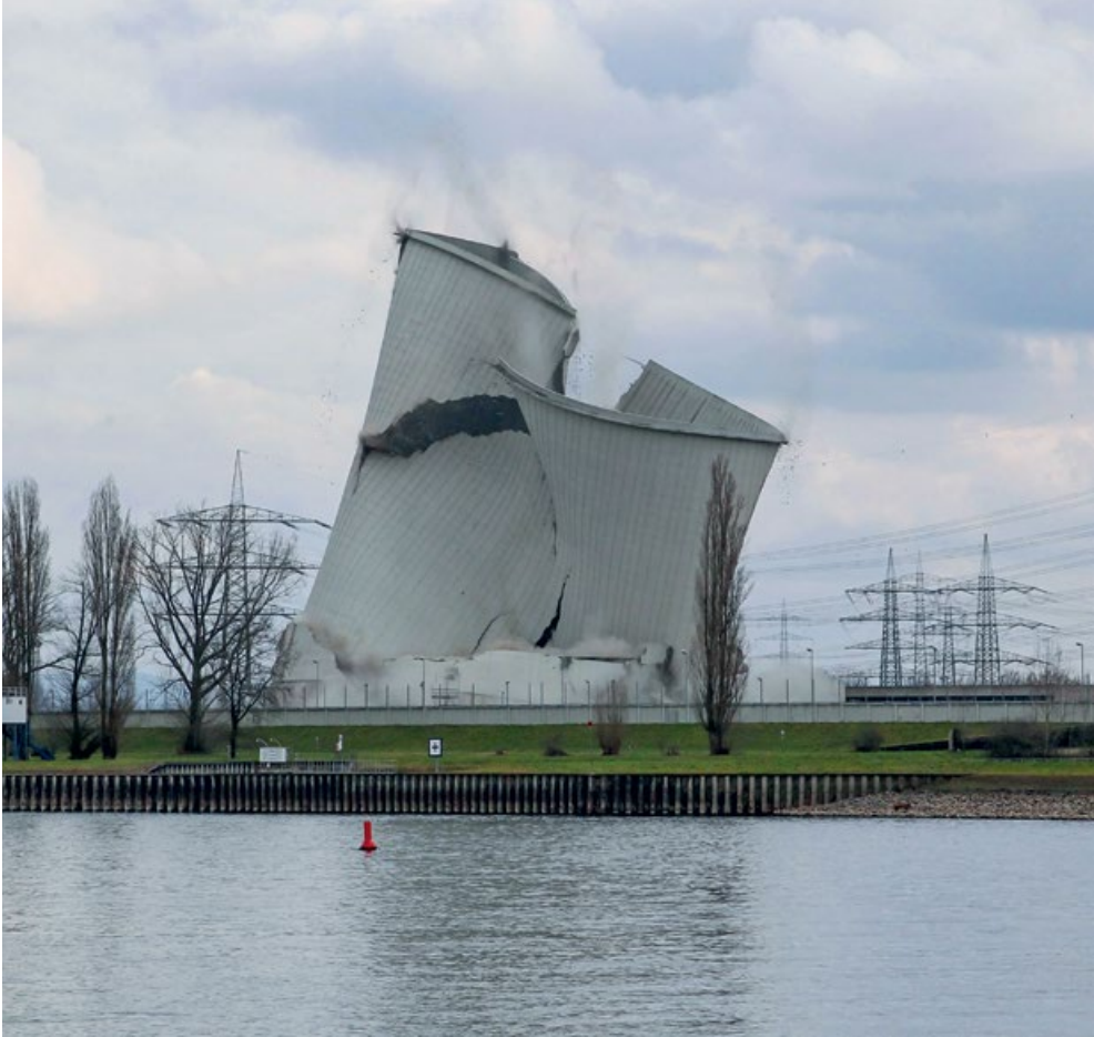
← Controlled demolition of the cooling tower at Germany's Biblis power plant (February 2023). After Fukushima, Berlin decided to phase out nuclear power and has been dismantling its reactors ever since.
